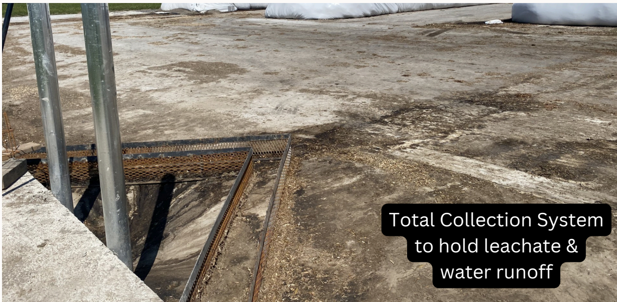
Concrete Curb & Apron to direct leachate
