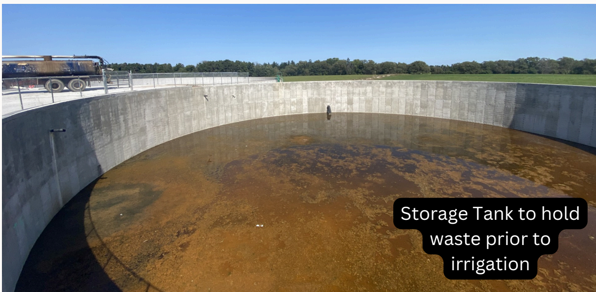
Total Collection System to hold leachate & water runoff
