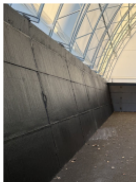
New Sealed Concrete Sides
